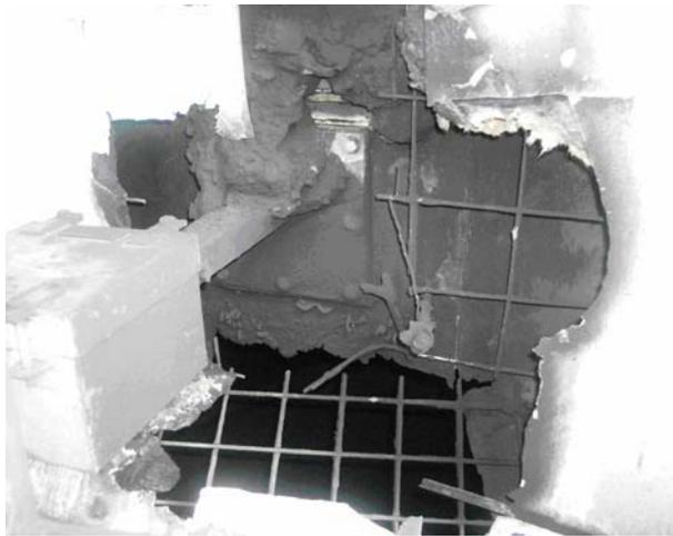
Figure 6. Chimney wall corrosion of unit -2 at (ZTPS) (15-7-2008)
