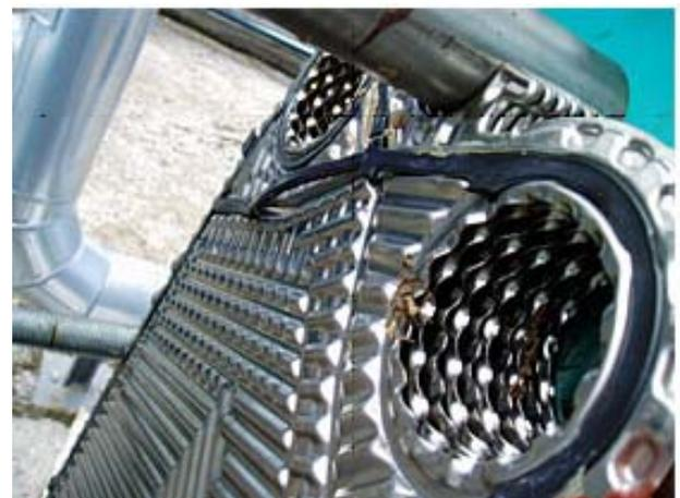
Picture 6 Cleaned warmth exchanging surface of the warmth exchanger
