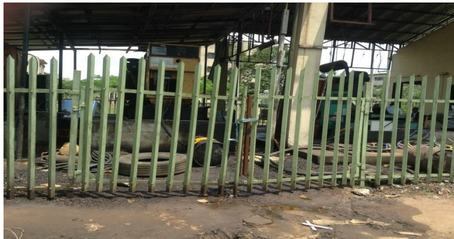
Figure 4 Pollution around the power house behind Dorcas Hall
