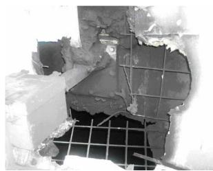
Figure 6.Chimney wall corrosion of unit -2 at (ZTPS) (15-7-2008)
