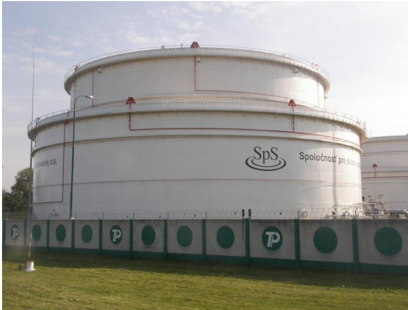
Figure 3. Storage tank with a capacity of 30,000 m 3 [8]
